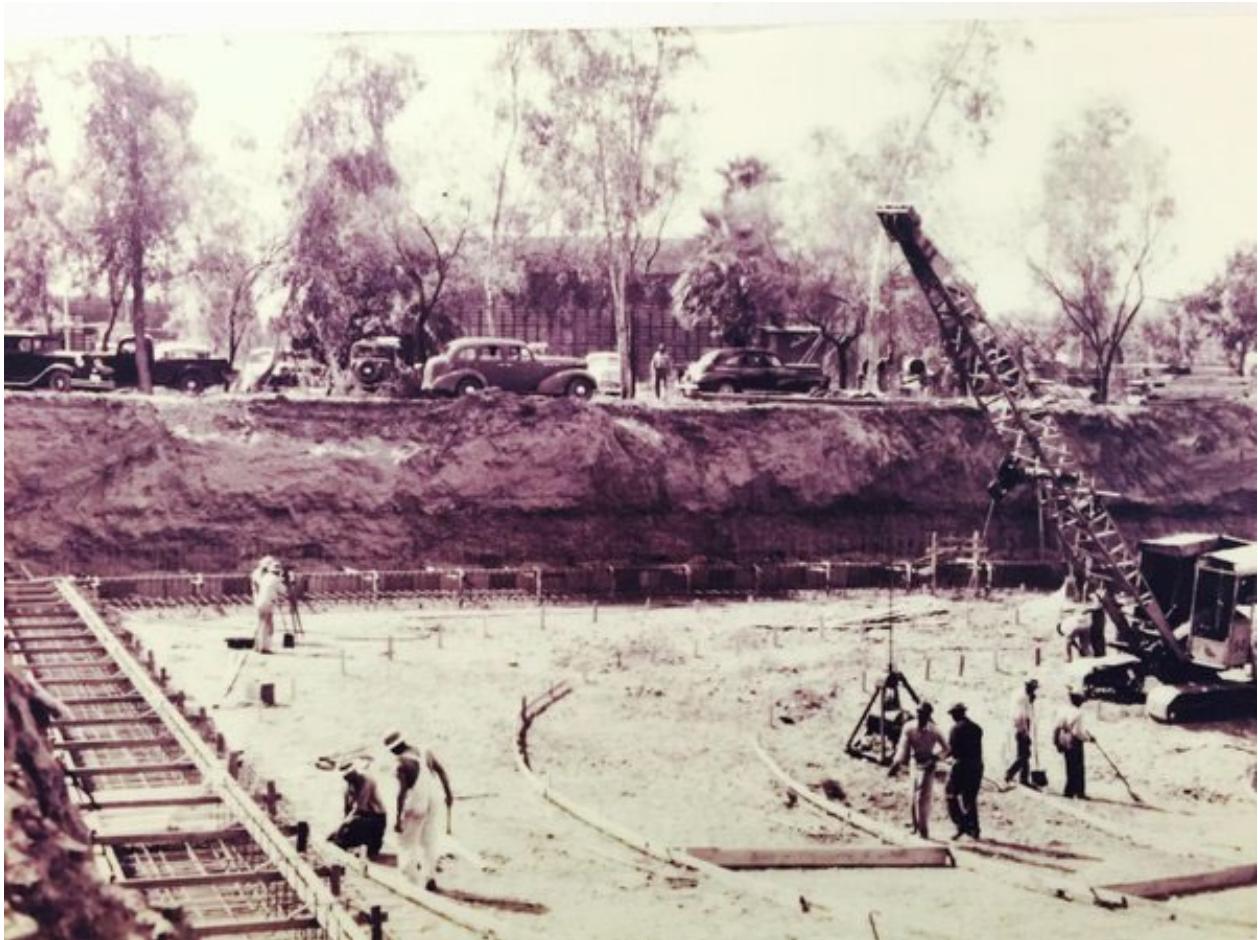
1947 Construction of Clarifier at 23rd Avenue WWTP
