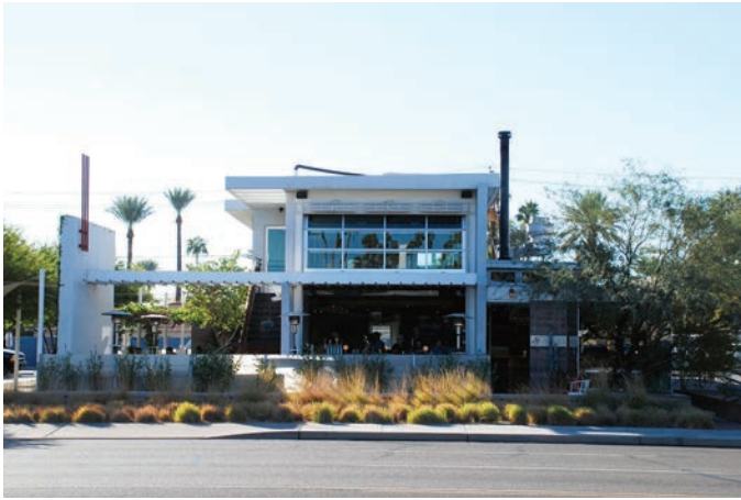
Adaptive Reuse - St. Francis Restaurant
