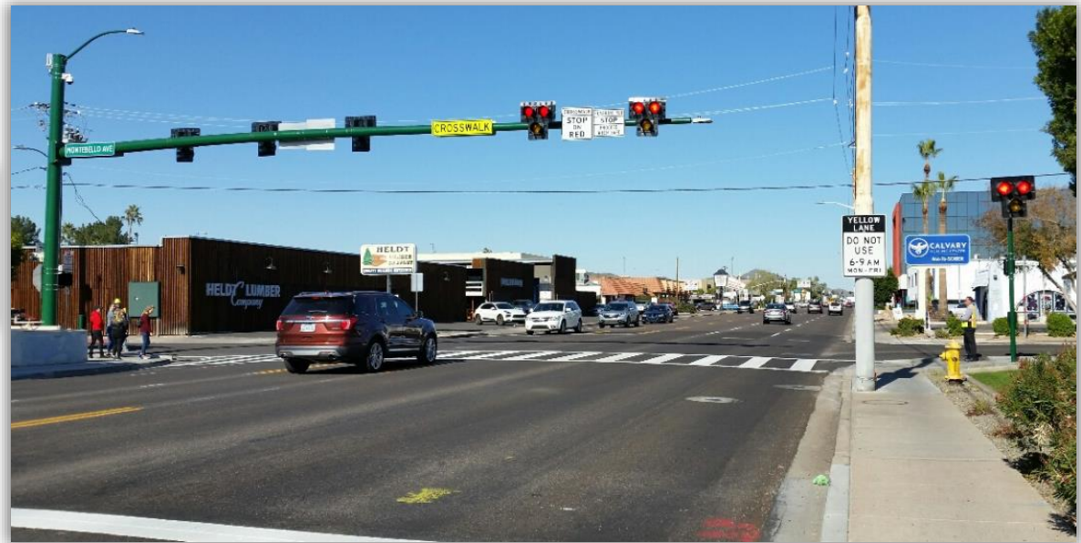
Pedestrian signal (HAWK) at the 7th Street and Montebello Avenue intersection.
