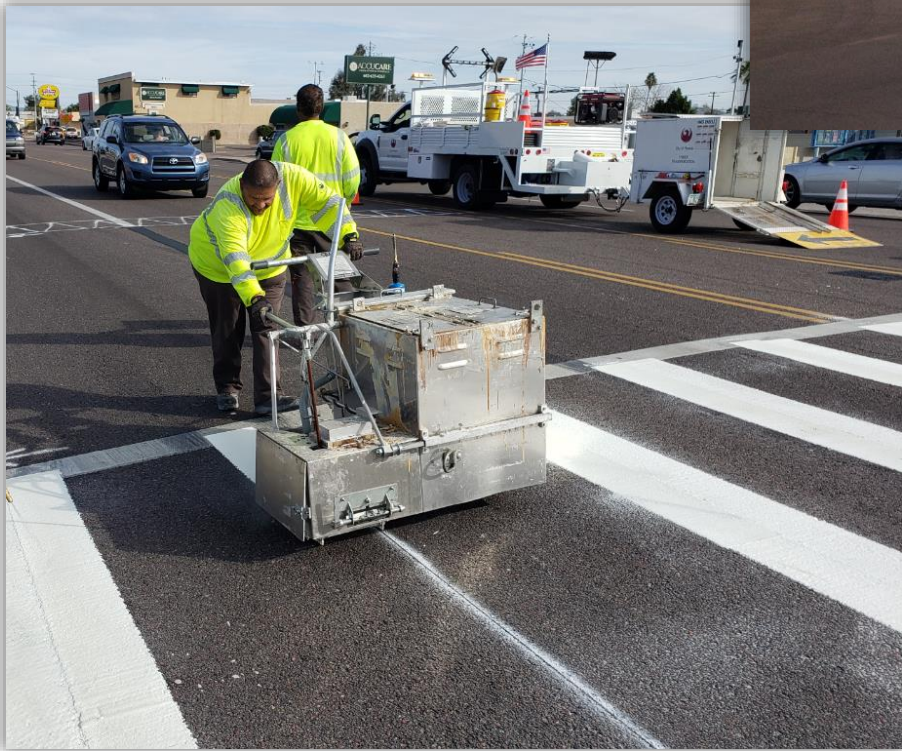
Crosswalk Upgrade Installation at 19 th Avenue and Fairmount Avenue.
