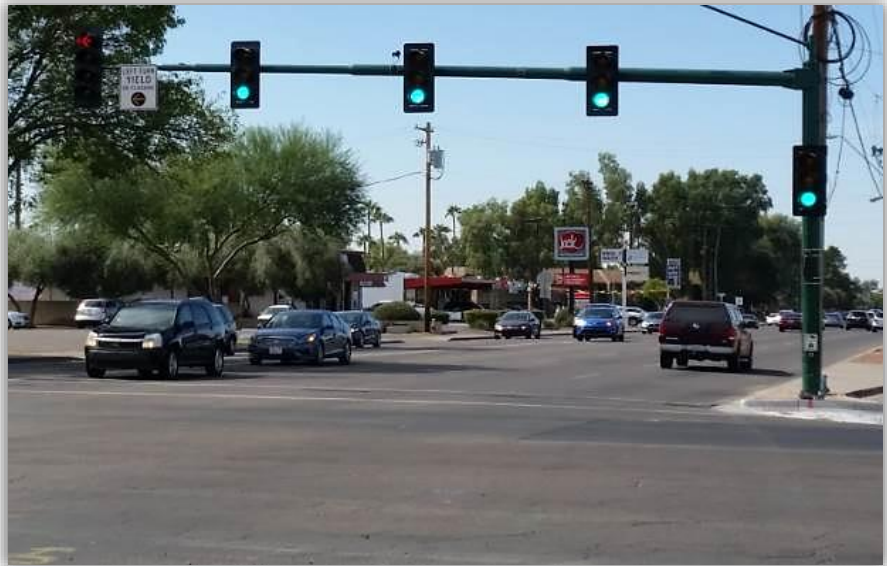
Traffic Signal Flashing Yellow Arrow and Pedestrian timing modifications at 12th Street and Northern Avenue.
