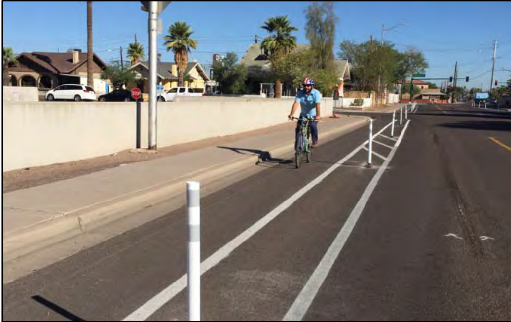
Protected Bike lanes on 15th Avenue from Jefferson to Van Buren Streets
