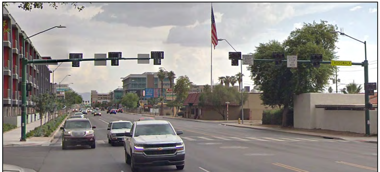
Pedestrian signal (HAWK) at the 7th Avenue and Fillmore Street intersection.
