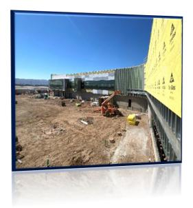
Terminal 4 Eighth Concourse construction work continues. Building work is ongoing with interior framing and exterior glazing. Interior work will consist of drywall installation, shaft wall framing, hearing loop installation and overhead and inwall utilities. Concourse permanent power is anticipated to complete by early May 2021.
